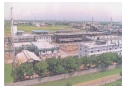
Suryapet, Telangana, India SUVEN Intermediate Mfg. Facility
