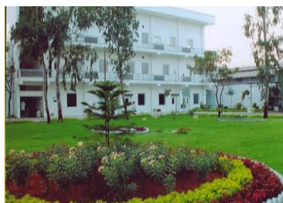
Jeedimetla, Telangana, India SUVEN R&D–Pilot Plant
