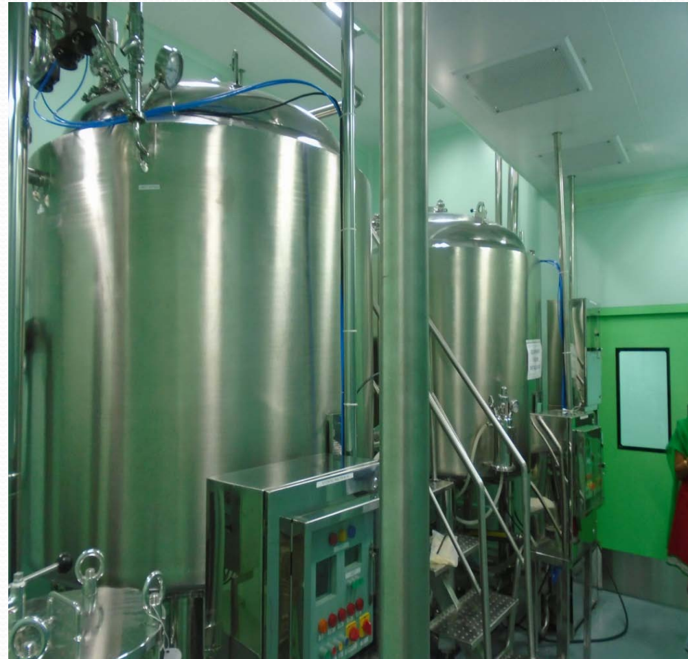
2000L Mixing Tank and 2000L Holding Tank
