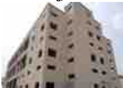
Multi-product/specialty chemicals facility Vizag, India
